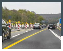
Visa-Line / FOL Temporary Pavement Marking Tapes are a highly economical solution when short-term temporary pavement markings are needed for construction or road repair. The pre-applied pressure sensitive adhesive on the conformable aluminum backing provides excellent bonding to most roadway surfaces. Just place on the roadway and tamp with your foot or a vehicle tire is all that is needed to apply to surface. Removal is just as easy - simply pull up the tape, leaving a clean surface underneath.
