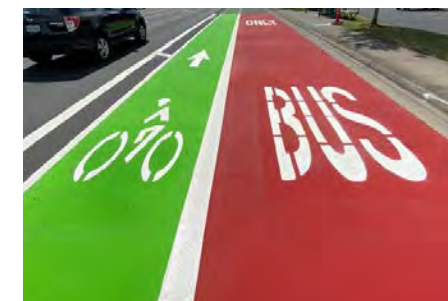
MMA Green Bike Lane & Red Bus Lane Markings
