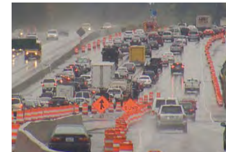
Construction Zone Markings
