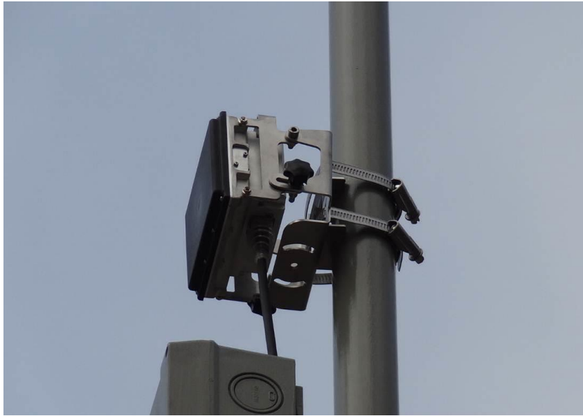
Figure 5: Bracket attached to pole using straps.
