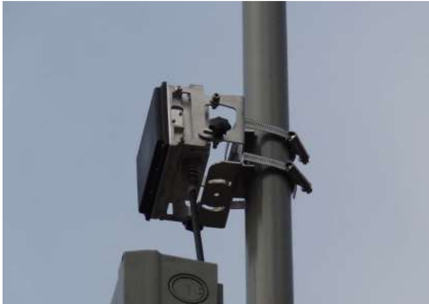
Figure 5: Bracket attached to pole using straps.
