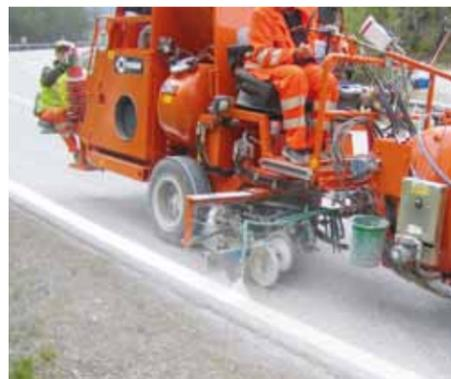
The standard system for secondary road networks: So-called type-I markings are a widespread and very cost-effective form of marking in many European countries.
