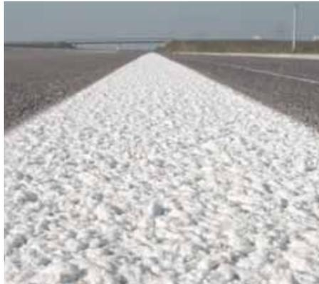
The structure makes the difference: Type II agglomerate markings with a structured surface deflect the wet better than any other system.
