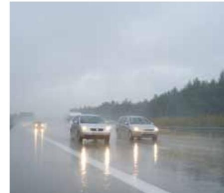
State of the art in modern marking systems: So-called type-II markings also demonstrate their visible strength at night on wet roads. Compared to type I, this means ever greater traffic safety, particularly on motorways.
