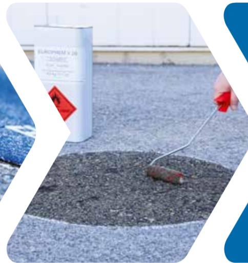
Preheat and/or pre-dry the substrate if it is cold or wet. Apply the primer and let it dry.
