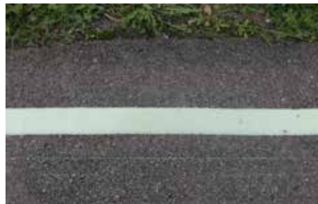
2-component afterglow plastic as edge line
