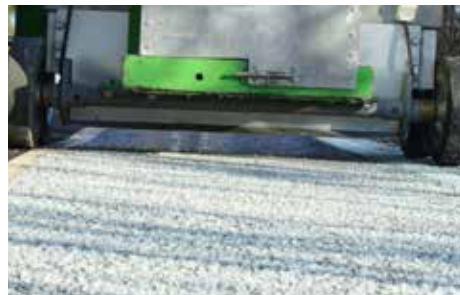
2-component afterglow plastic as edge line combined with 2-component cold plastic (transparent) with drop-on afterglow aggregates mix
