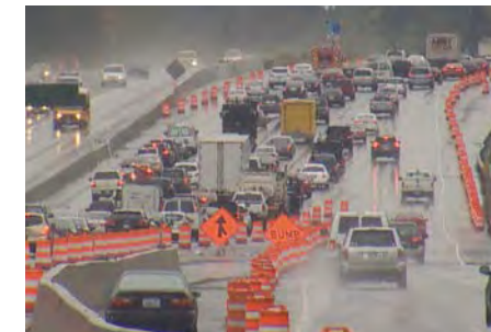
Construction Zone Markings
