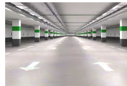
Parking Garage Markings
