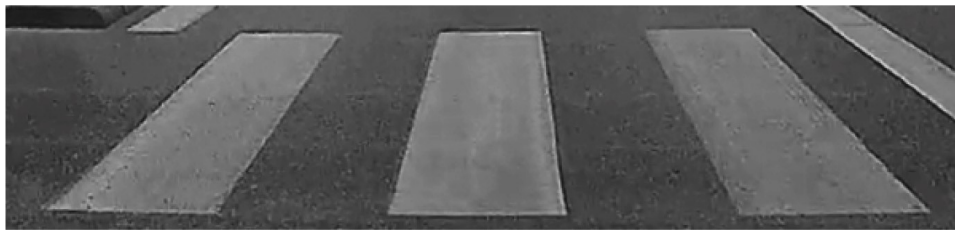
Fig. 1. Exemplary area (crossing B) at the beginning of analysis: circa 2% marking loss since last application (period on the road unknown).
