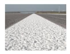
The structure makes the difference: Type II agglomerate markings with a structured surface deflect the wet better than any other system.
