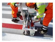
The standard system for secondary road networks: So-called type-I markings are a widespread and very cost-effective form of marking in many European countries.
