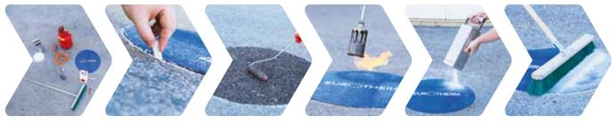
Equipment: gas torch, broom, piece of chalk, and drop-on beads; primer only if necessary The area to be marked must be completely clean, dry and free of dust and oil. Draw the outline in chalk If it is cool and moist, preheat and dry the substrate. Apply primer and let it flash off. Use a gas torch to heat the entire surface of the EUROTHERM marking until it starts to bubble.
