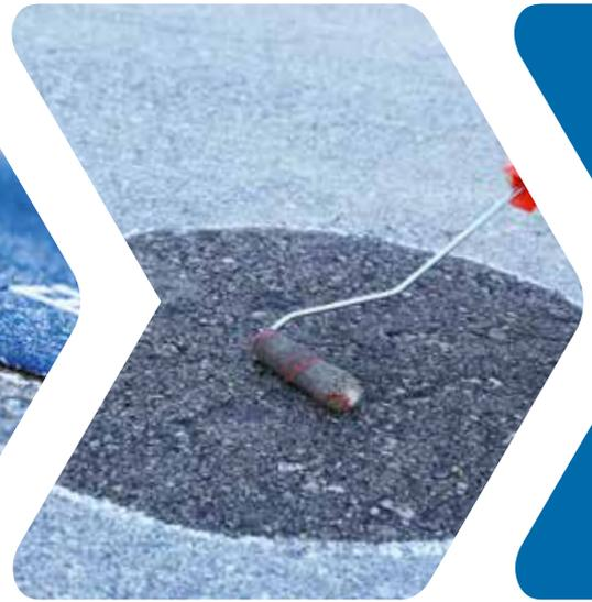
If it is cool and moist, pre-heat (thoroughly dry) the substrate. If necessary, apply primer and let it flash off.
