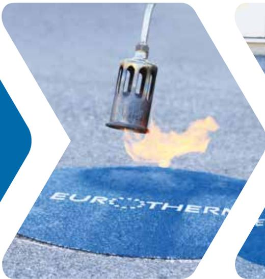
Use the torch to heat the entire surface of the EUROTHERM until it starts to bubble.
