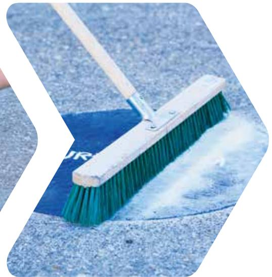
Use the broom to clean the EUROTHERM and use a sharp object to check that it is securely adhered. The marking can be driven over after just a few minutes.
