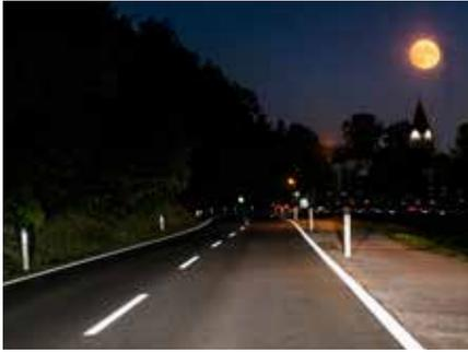
State of the art in modern marking systems: So-called type-II markings also demonstrate their visible strength at night on wet roads. Compared to type I, this means ever greater traffic safety, particularly on motorways.
