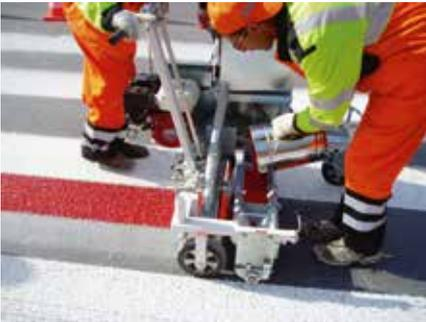
The standard system for secondary road networks: So-called type-I markings are a widespread and very cost-effective form of marking in many European countries.
